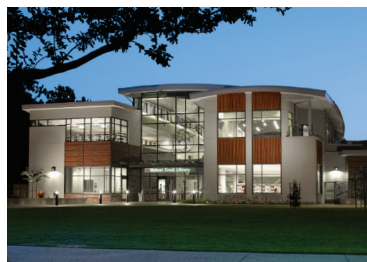
Walnut Creek Library, Walnut Creek CA Group 4
